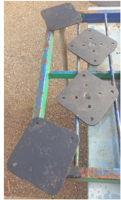
Plates & legs ready for footings for shade structure
