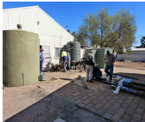
Shade structure gone & assembling new Aluminium structure
