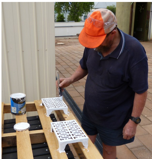
Col painting a pair of cast air vents
