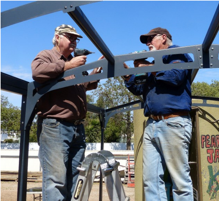
Riggers Rob & Jim assembling shade structure rear of hall
