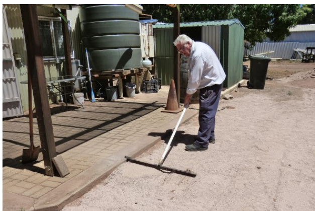
Andy grading the sand for the laying of the pavers
