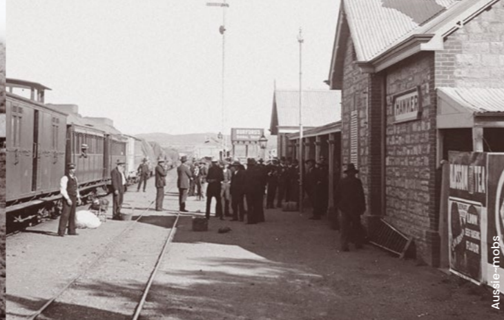
11 Hawker Railway Station, approximately 1908
