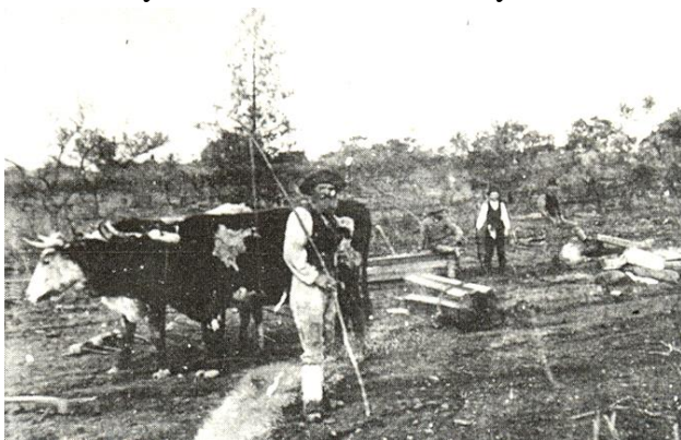
Cutting railway sleepers by the Warrioota Creek. Looks as if the bullock team will haul them along the ground itself
