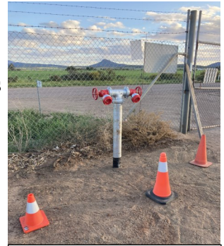
One of the new fire hydrants at the Quorn Depot
