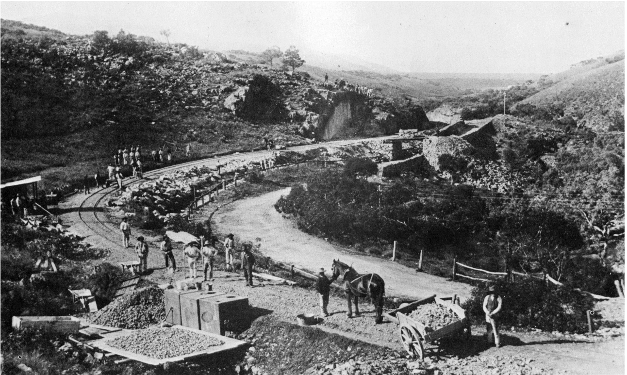
Work commencing on new cuttings to ease some of the sharper curves in 1888
