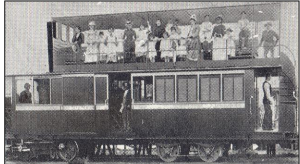
1884 double-deck Country Steam Motor, built in Belgium for SAR. Vertical boiler at front. Rolled tarp at the left end?
