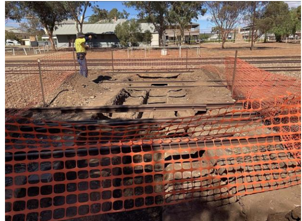
Culvert 0 exposed across depot tracks
