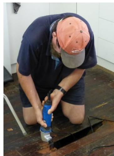
Col repairing a broken board in kitchen floor
