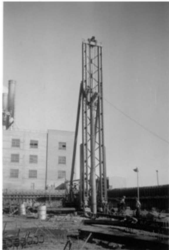
Franke Pile Frame Driver 'B' Station
