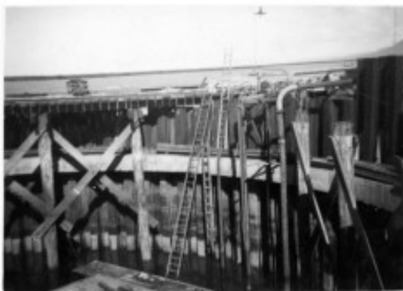
Inside view of Coffor Dam pump House site
