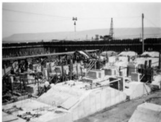
Footings poured Photo by George Jamieson
