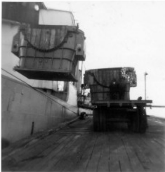
Turbine Block being unloaded from the Belnor at the Power House Wharf
