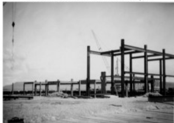
Erecting Steel for 'B' Station
