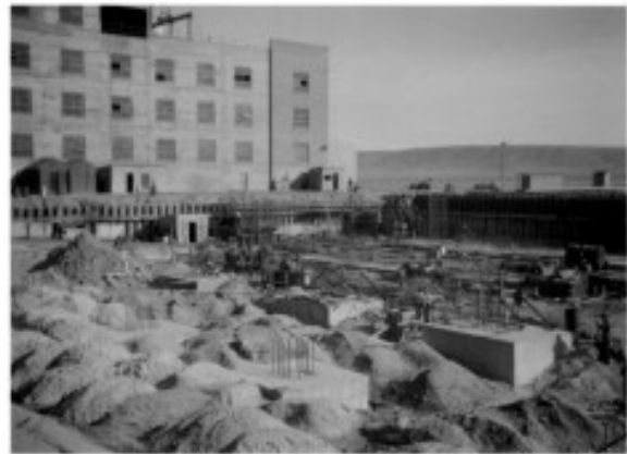
'B' Station Footings
