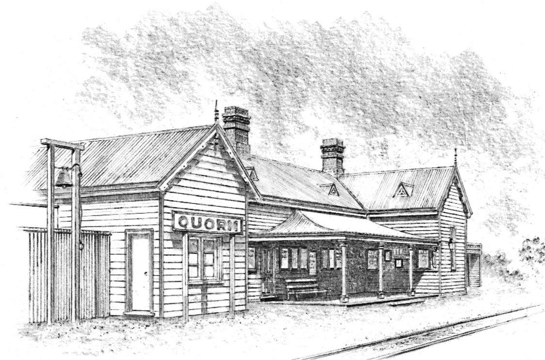
The original timber station building stood between the present building and the tracks, where there is now a wide platform area
