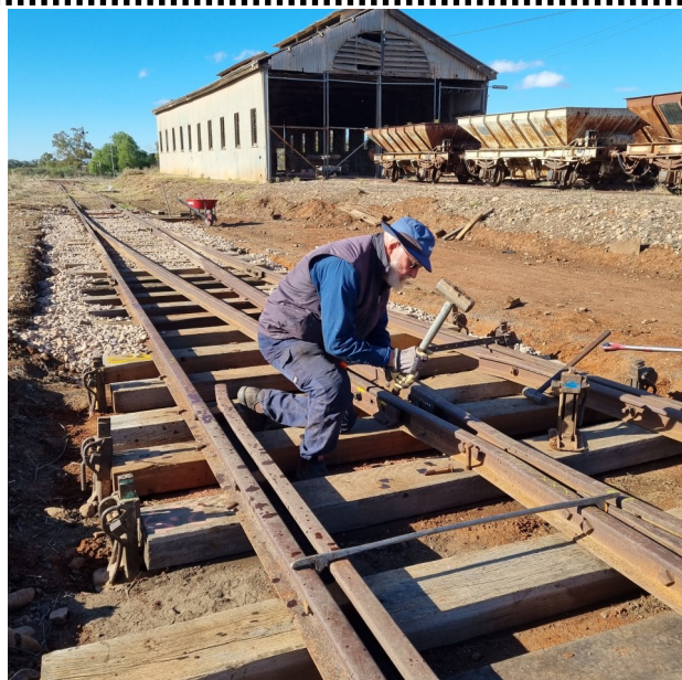
Volunteer John Humphries hammering in dog spikes to secure the track to sleepers at the rebuild of the old railway line "turn-out" (where the track splits into two lines). This picture depicts the rails behind being supported by new wooden sleepers embedded in rock ballast, while a "gauge bar" in the foreground keeps the track gauge at precisely 3 foot 6 inches or narrow gauge. In the background can be seen the old SAR Engine Shed, Quorn
